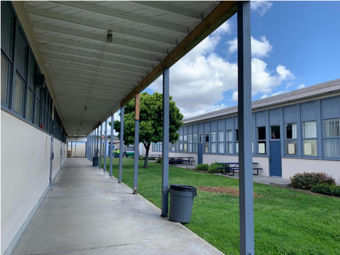
Existing Walkway Post
